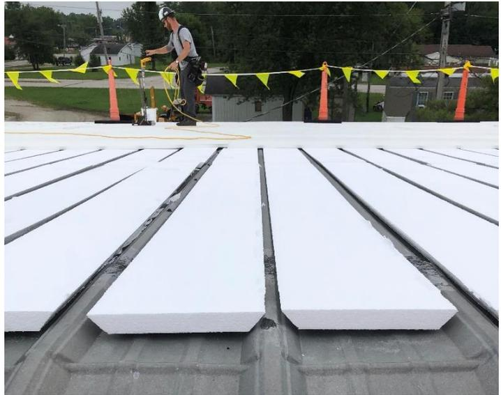
*Cellofoam Flute Fill in the foreground. In the background, a roofer is installing Cellofoam FR Composite Sheet over the flute fill.*
