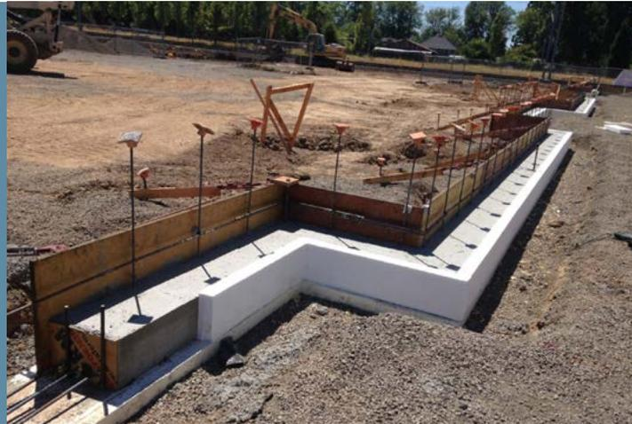
The Expanded Polystyrene Association of Canada (EPAC) conducted a joint research project with the National Research Council of Canada/ Institute for Research in Construction (NRC/ IRC) to evaluate the durability performance of expanded polystyrene (EPS) insulation in an exterior below-grade application.<sup>1</sup> EPS insulation, thermal performance, site weather conditions and soil moisture content were instrumented and monitored throughout the project.
